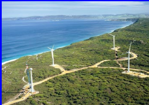
Albany wind farm, W.A.
